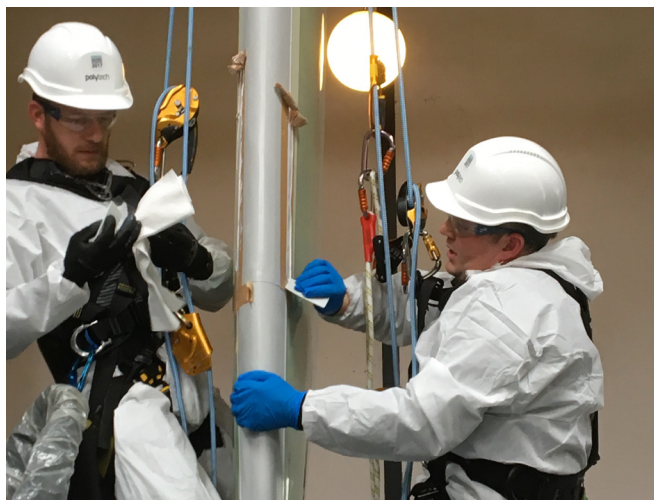
The application of ELLE involves no chemical hazards and generates no hazardous waste.
